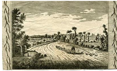
The Great North Road near Highgate on the approach to London before turnpiking. The highway was deeply rutted and spread onto adjoining land.
